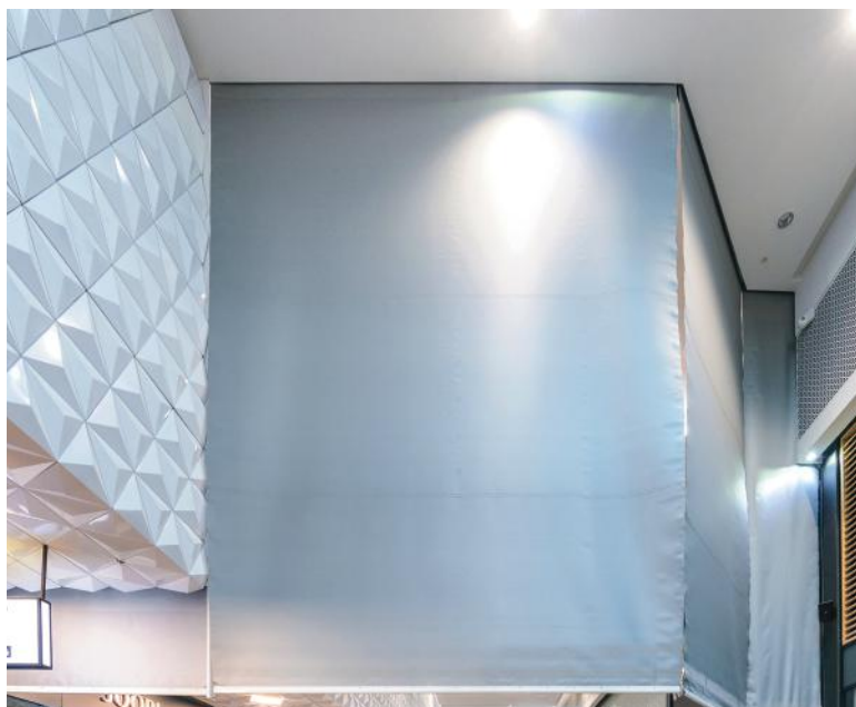
Fig. 41 – mcr PROSMOKE material smoke curtain
