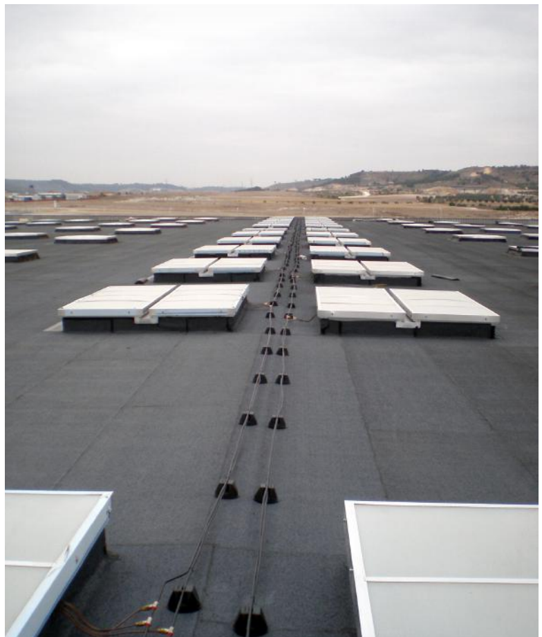
Fig. 6 – mcr PROLIGHT double leaf smoke vents
